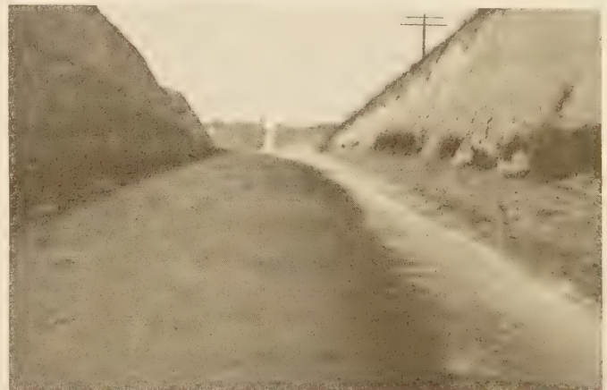
FIG. 2.—Location of the road over the loess formation and the steep angle of repose of this type of soil
